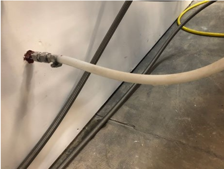
Vacuum pump hose( 1/2" braided silicone hose) coming into DR-10 room
